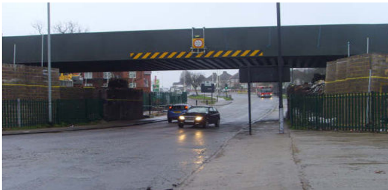
The new bridge as it stands today.
