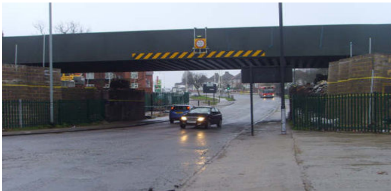
The new bridge as it stands today.
